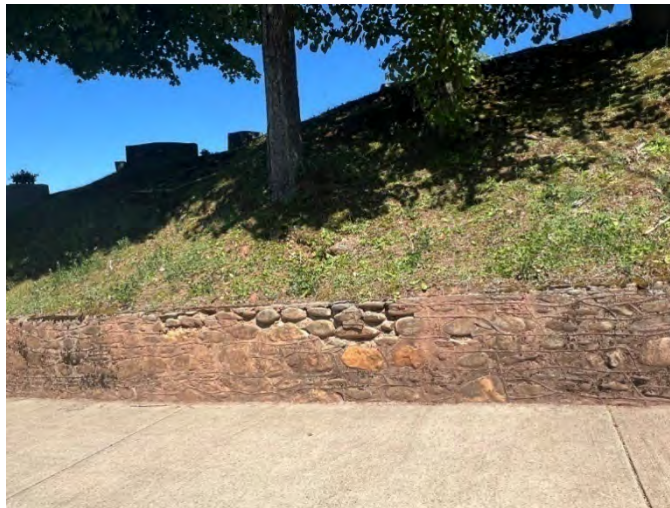
Figure III.4. View east of the retaining wall along Hillview Circle, showing mortar loss and organic growth.
