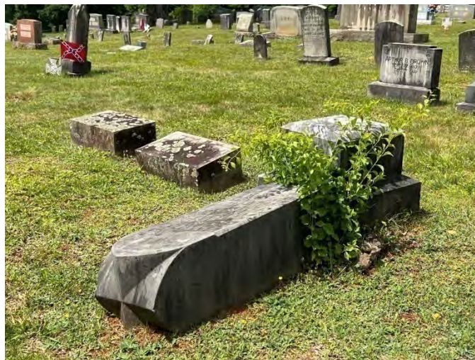
Figure III.32. The shaft of this marble pedestal tomb with vaulted roof is displaced from its stacked bases.
