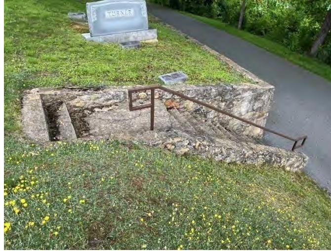
Figure III.15. Stairs leading from the upper level of the cemetery to Veterans Circle, showing moss and debris collected in the upper corners.
