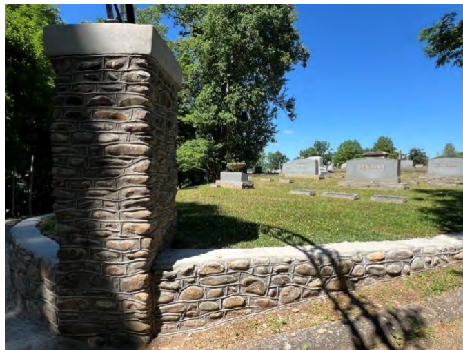
Figure III.2. View north of the recently completed masonry restoration of the stone piers and retaining walls at the main entrance.
