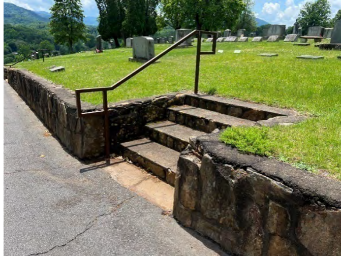
Figure III.13. View southwest of steps and retaining walls at the northeast corner of Veterans Circle, showing asphalt applied to the top of the wall.
