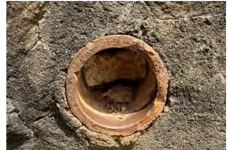
Clogged Weephole in Retaining Wall
