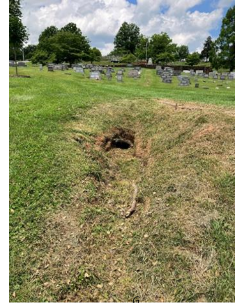
Crushed Outfall Pipe
