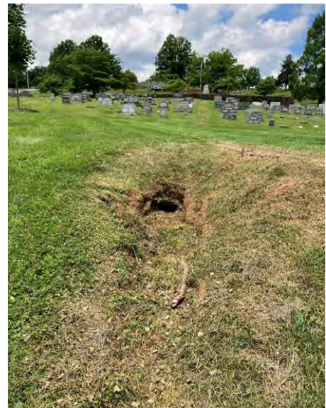
Crushed Outfall Pipe
