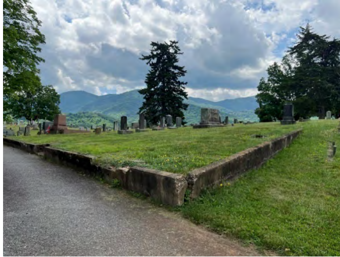
Figure III.9. View southeast of a low concrete retaining wall that is cracked and failing.
