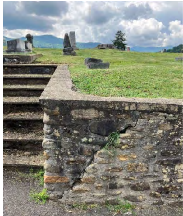
Cracks in Retaining Wall
