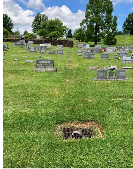
Grated Yard Inlet Downstream of a Swale
