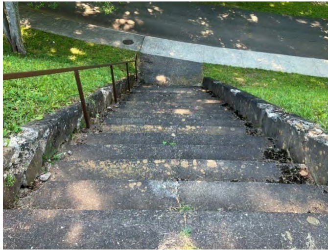
Figure III.5. View west of steps leading to Hillview Circle, showing lichen, moss, and spalling concrete.
