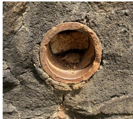
Clogged Weephole in Retaining Wall
