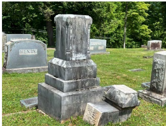
Figure III.34. This square column is also broken and needs to be cleaned and repaired.
