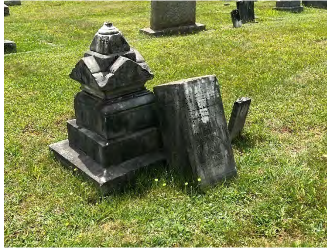
Figure III.33. This square column is broken down into three or four parts and is covered with a dark film of atmospheric staining and biofilms.
