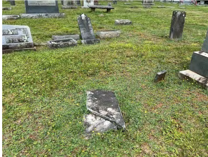
Figure III.25. A marble tablet that has broken and fallen from its upright position.
